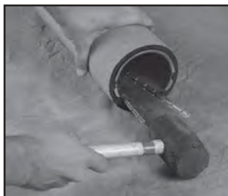
Figure 19 Install Split Ring Stiffener in PE pipe
