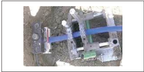
Fig. 12 Service Butt Fusion
