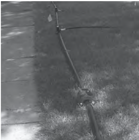
Figure 19 Example of Above Ground PE Bypass Pipe
