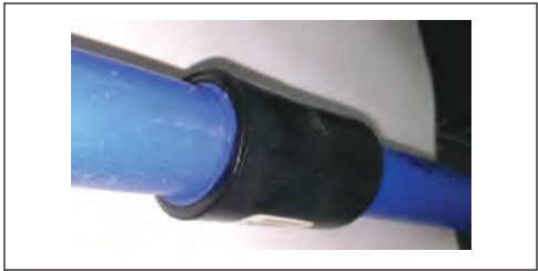
Fig. 13 Service Line Socket Fusion
