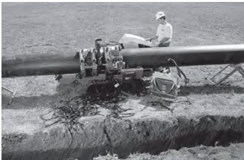
Figure 1 Above Ground Repair with Fusion Machine
