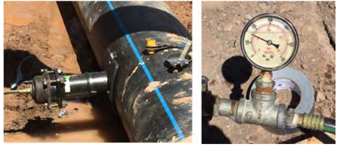
Figure X-p – Pressure Testing
