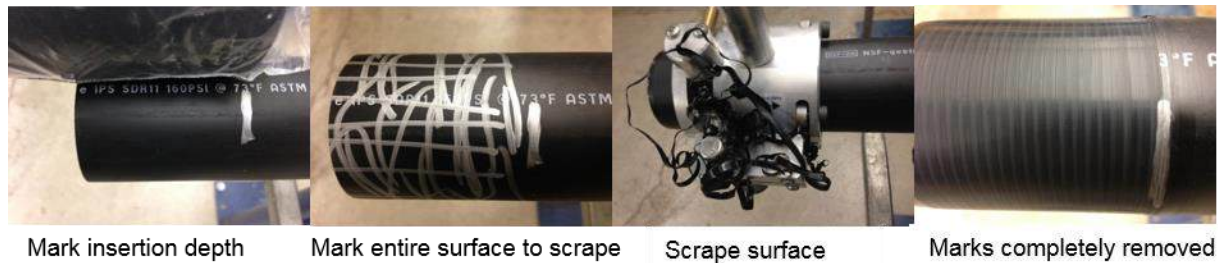
Figure X-o - Correct Scraping
