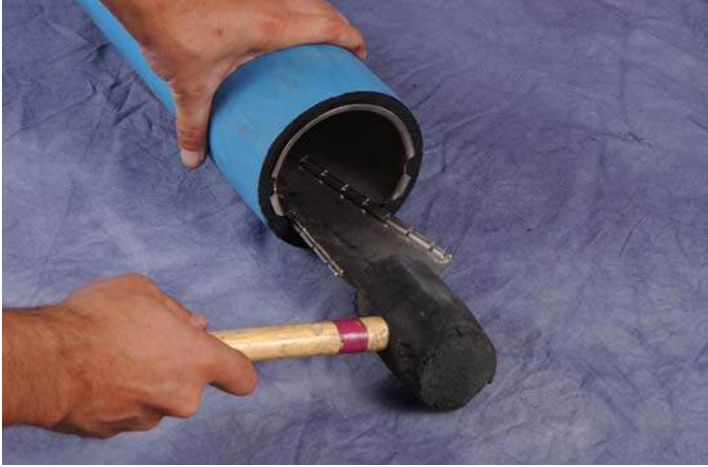
Figure 23 Install Split Ring Stiffener in HDPE pipe
