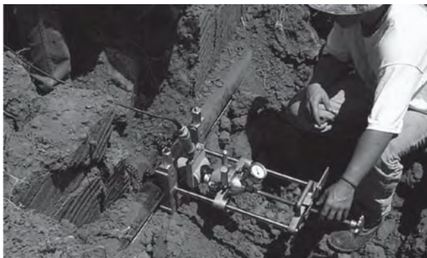
Figure 3 Saddle Fusion Repair
