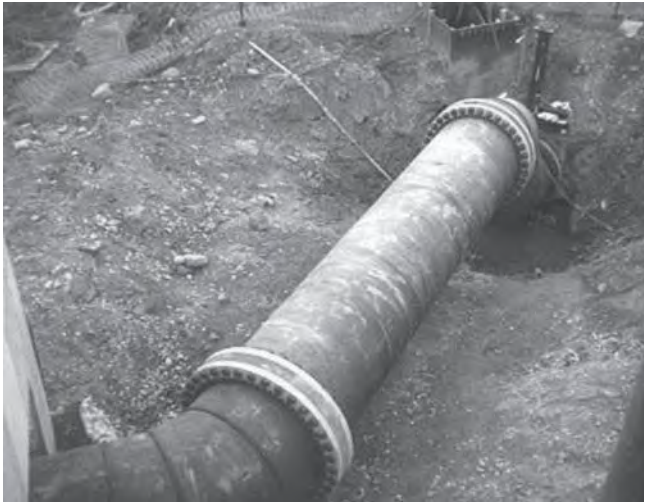
Figure 13 Flange Adapter Assembly
