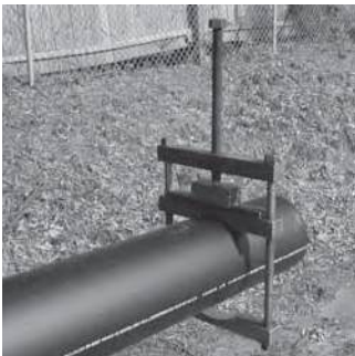
Figure 15 Mechanical Re-Rounding Clamp Installed
