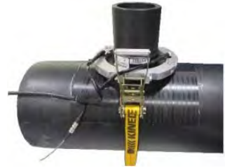
Figure X-n – Place Saddle Over Scraped Surface
