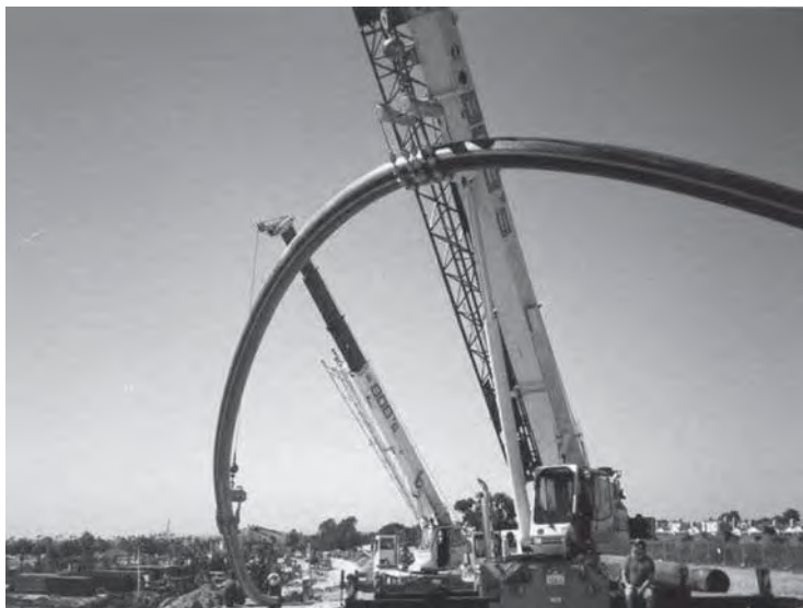
Figure 3 Butt Fused PE Pipe “Arched” for Insertion into Directional Drilling Installation
