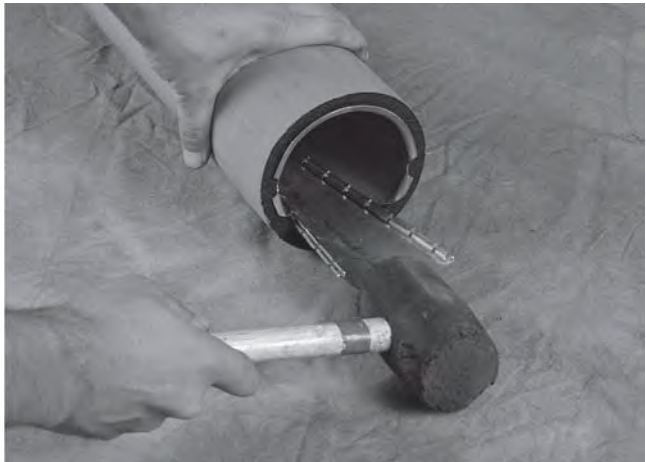
Figure 12 Install Split Ring Stiffener in PE Pipe
