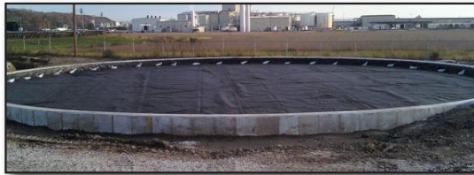
Secondary Containment - Installation of HDPE ringwall liner in a petrochemical facility.
