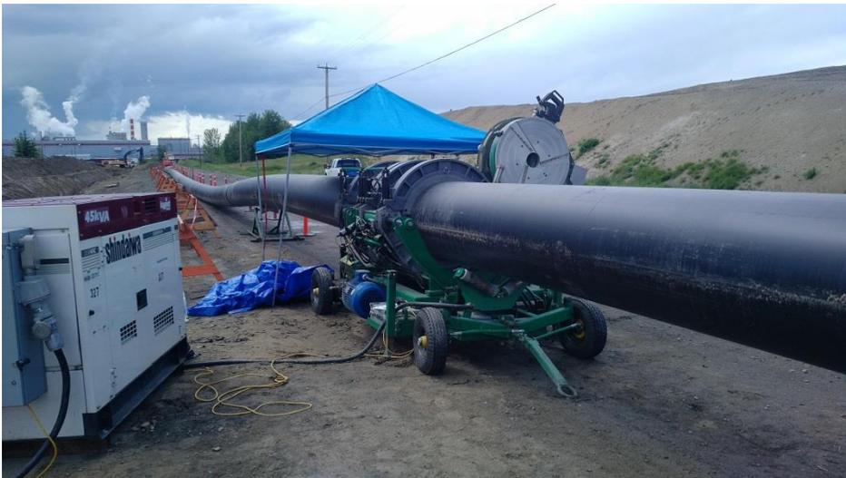
**Photo 4: Shows Heat Fused Joint of PE-RT Pipe**
